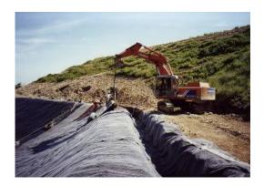
The end of the liner should be placed into the anchor trench when the roll is being situated on the slope. Once the liner is in position the end of the liner should be down the side of the anchor trench and across the bottom, do not bring the liner up the other side of the anchor trench as this configuration would water reduce hold and the effectiveness of the anchor trench. Any excess liner should be folded in the bottom of the trench.
