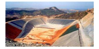
GCL to reinforce the system, if necessary.
