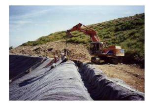
The end of the liner should be placed into the anchor trench when the roll is being situated on the slope. Once the liner is in position the end of the liner should be down the side of the anchor trench and across the bottom, do not bring the liner up the other side of the anchor trench as this configuration would hold water and reduce the effectiveness of the anchor trench. Any excess liner should be folded in the bottom of the trench.
