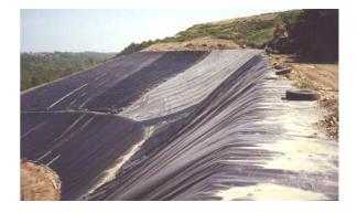
Exceptionally, a thickness of less than 0.5 m may be applied in projects involving special solutions for the execution of the sidewall containment barrier system, which in any case must guarantee the same level of protection. This can be achieved easily by using a geosynthetic clay barriers either singly or in pairs.
