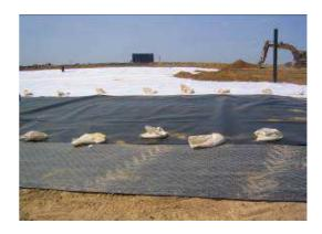
The GCL can therefore stand in place with the only cover being the flexible membrane. During construction of the landfill liner the GCL should not remain uncovered by the flexible membrane for any longer than is necessary, and should not be laid too far ahead of the flexible membrane.
