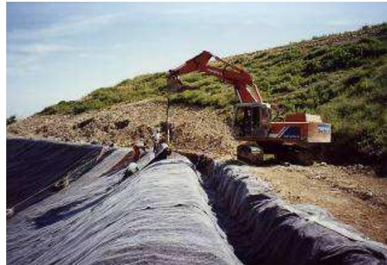
The end of the liner should be placed into the anchor trench when the roll is being situated on the slope. Once the liner is in position the end of the liner should be down the side of the anchor trench and across the bottom, do not bring the liner up the other side of the anchor trench as this configuration would hold water and reduce the effectiveness of the anchor trench. Any excess liner should be folded in the bottom of the trench.
