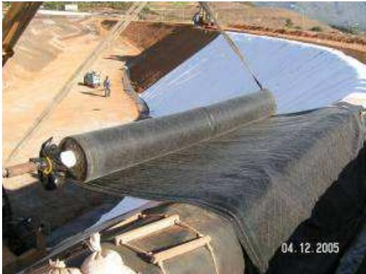
When Modulo Geobent XP is being placed on a steep slope it might be more convenient to attach the end of the GCL in the anchor trench and roll the GCL down the slope by passing a lifting pipe through the core of the roll attach a rope at each end and ease the roll down the slope by hand, instead of pulling the liner off the supporting bar, this is always difficult if the slope is too steep.
