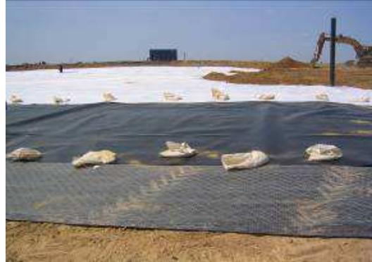
The GCL can therefore stand in place with the only cover being the flexible membrane. During construction of the landfill liner the GCL should not remain uncovered by the flexible membrane for any longer than is necessary, and should not be laid too far ahead of the flexible membrane.
