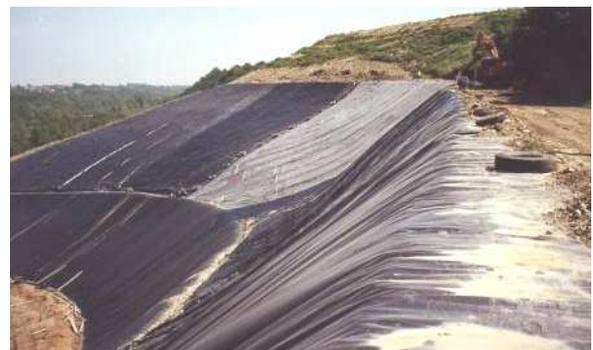
Exceptionally, a thickness of less than 0.5 m may be applied in projects involving special solutions for the execution of the sidewall containment barrier system, which in any case must guarantee the same level of protection. This can be achieved easily by using a geosynthetic clay barriers either singly or in pairs.
