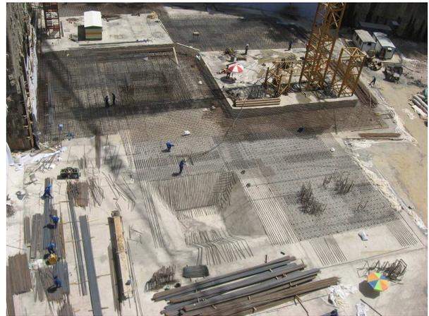
The reinforcing system of Edilmodulo XP makes a pre-confinement of the barrier and makes it useful especially for pre-casting applications (e.g. against diaphragm walls). It allows also the GCL capable of staying unconfined for a while without the final protection of the concrete layer.
